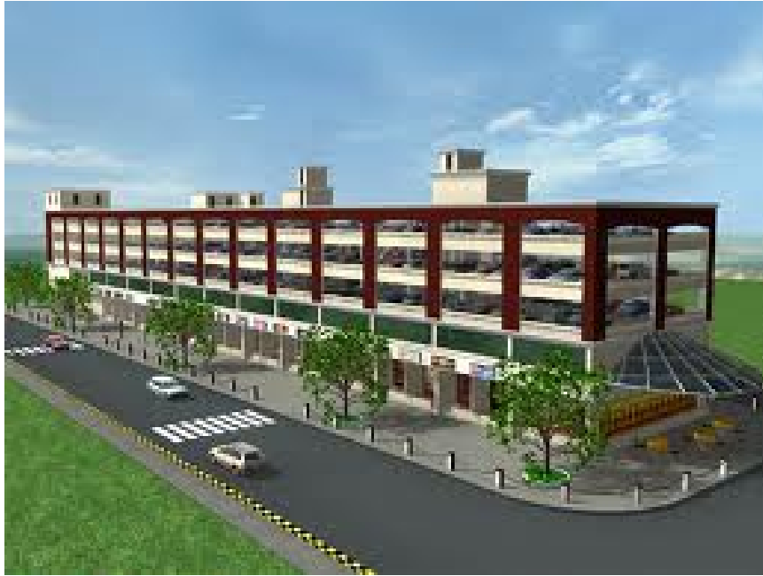
TYPICAL VIEW OF MULTI-LEVEL CAR PARK
